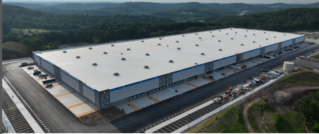
Amazon invested $120 million to build a 1 million-square-foot warehouse facility that is expected to create as many as 600 new jobs in New Stanton. Construction was completed in late 2023. Courtesy SunCap Property Group.
